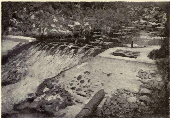
FIG. 3.—WEIR ON SMALL STREAM FOR HYDRO-ELECTRIC PLANT.
